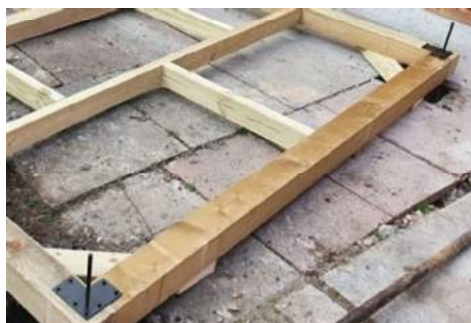
FIGURE D Eco Feet Part A installed
